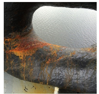
Poorly maintained deck equipment
