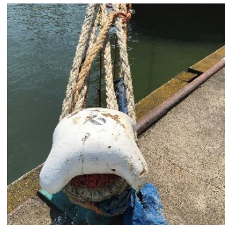
Mixed mooring not recommended and poor mooring plan
