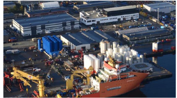
New warehouse and office, Dusavika base, Norway
