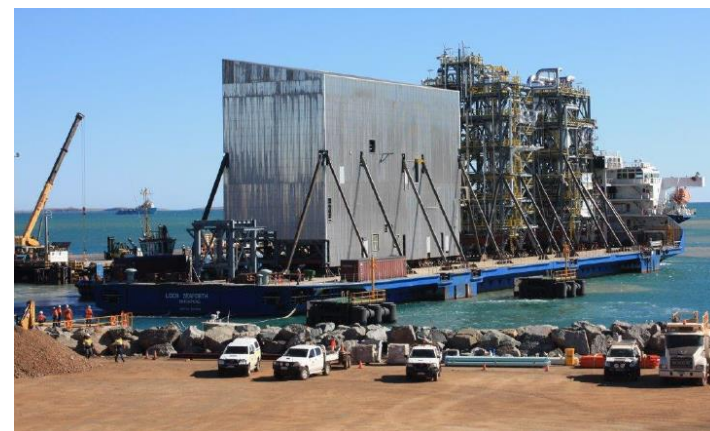
Heavy lift operation, Dampier, Western Australia Source: Qube
