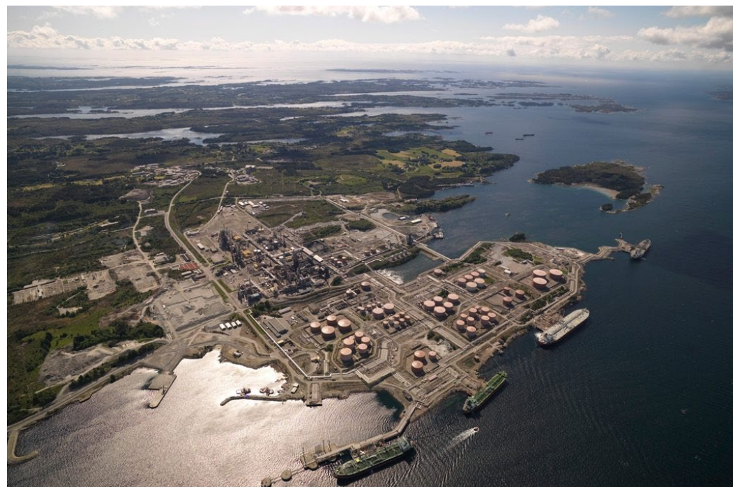
Mongstad Industrial Park has been selected as the location for what could become Norway's first production plant for liquid hydrogen serving the maritime market. Photo: Øyvind Hagen, Equinor Mongstad.
