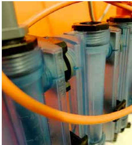
Sensors for condition monitoring of the boiler water.
