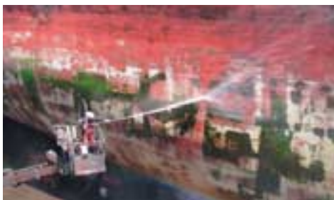
A fouled hull and propeller can increase vessel resistance in the water by 5-20%. During a docking, barnacles and other marine organisms are removed from the underwater hull and a new coat of tin-free antifouling applied.
